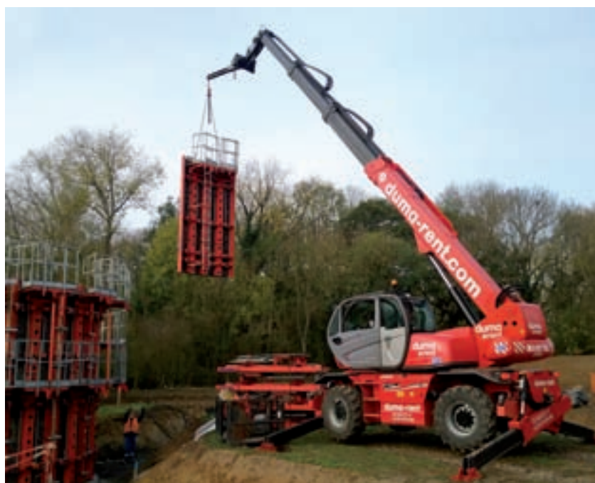
Duma @ Villereau (FR) / MANITOU MRT2550 + GIEK
