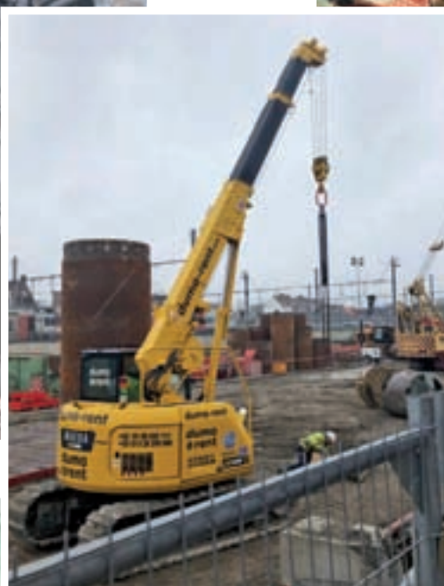
Maeda CC1485 construction d'un parking souterrain @Courtrai
